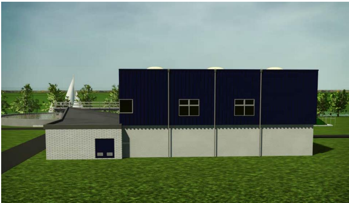
WwTW Franeker, Wetterskip Fryslân – tertiary filtration for P and N removal
