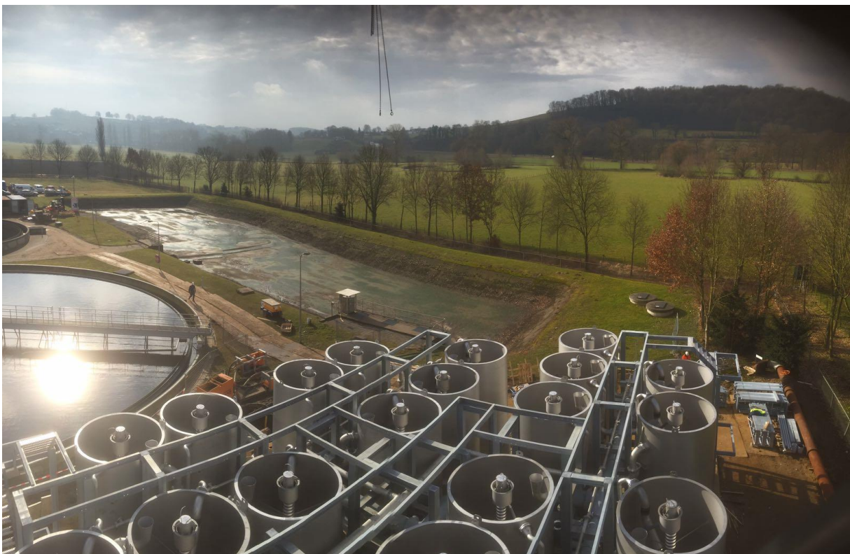
WwTW Wijlre, tertiary biofiltration for N and P removal
